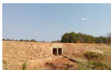
Km 38+000 on Link 2, after Re-instatement
