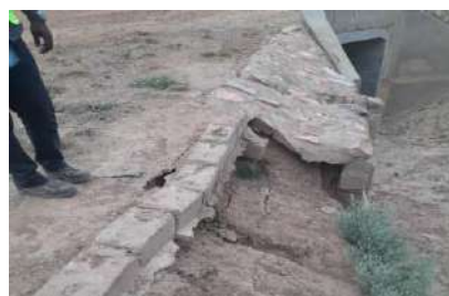
Left view of reinstated road at Km86
