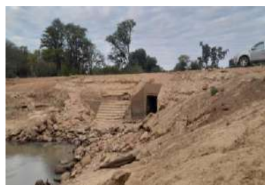
Reinstated road crossing on link 2
