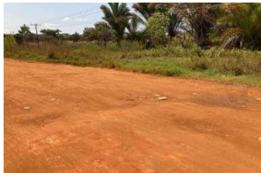
Part of the access road to Samora Machel Airport
