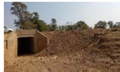
Km 86 + 000 On Link 2, after Re-instatement
